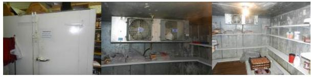
12'x10' Walk-In Cooler\* w/ Floor & Bohn Condenser/ Compressor\*
