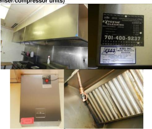
14'x48" Exhaust Fan w/ Heated Make-Up Air, Fire Suppression, Roof System, & Stainless Wall Panels (pricey unit!!)
